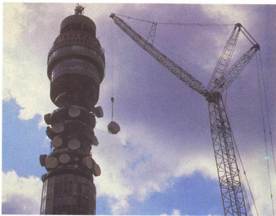
As seen on TV, British Telecom's changeover to a digital phone system proceeds apace. Here, a dish is hauled into position high up on the Telecom Tower.
